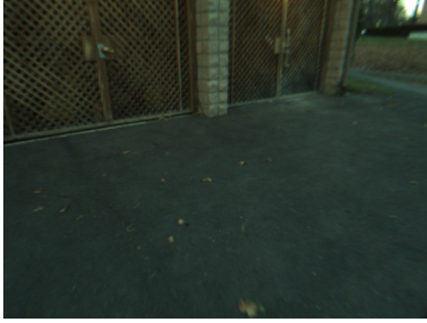
(a) Our garage wall.
